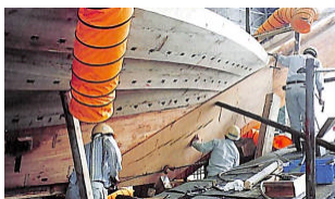
Fig.11 Forward shell structure called 'Yotoori'
