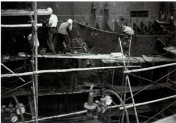
Fig.4 Bulge Construction of Soya
