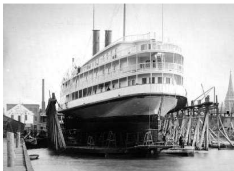
図1-13 Marine Railway型修船架
