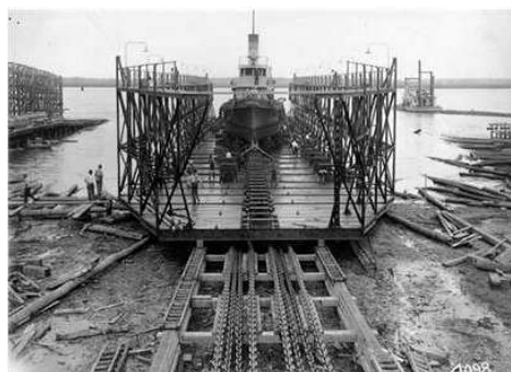
図1-14 Marine Railway改造型修船架
