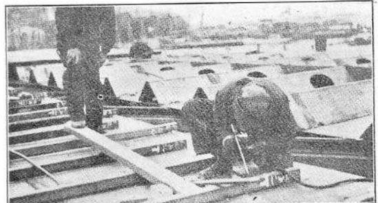
Stiffeners being Welded to Bulkhead. Bottom Plates with Frames and Side Keelson shown in the Background.
