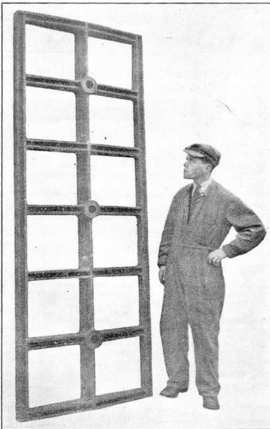
Fig. 5. Cast Monel Metal Pickling Raft, 8 ft. by 6 ft. overall.
