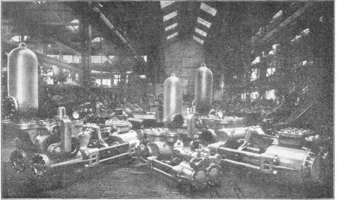
Group of Clarke, Chapman Cargo-oil Pumps supplied to Aktiebolaget Götaverken.
